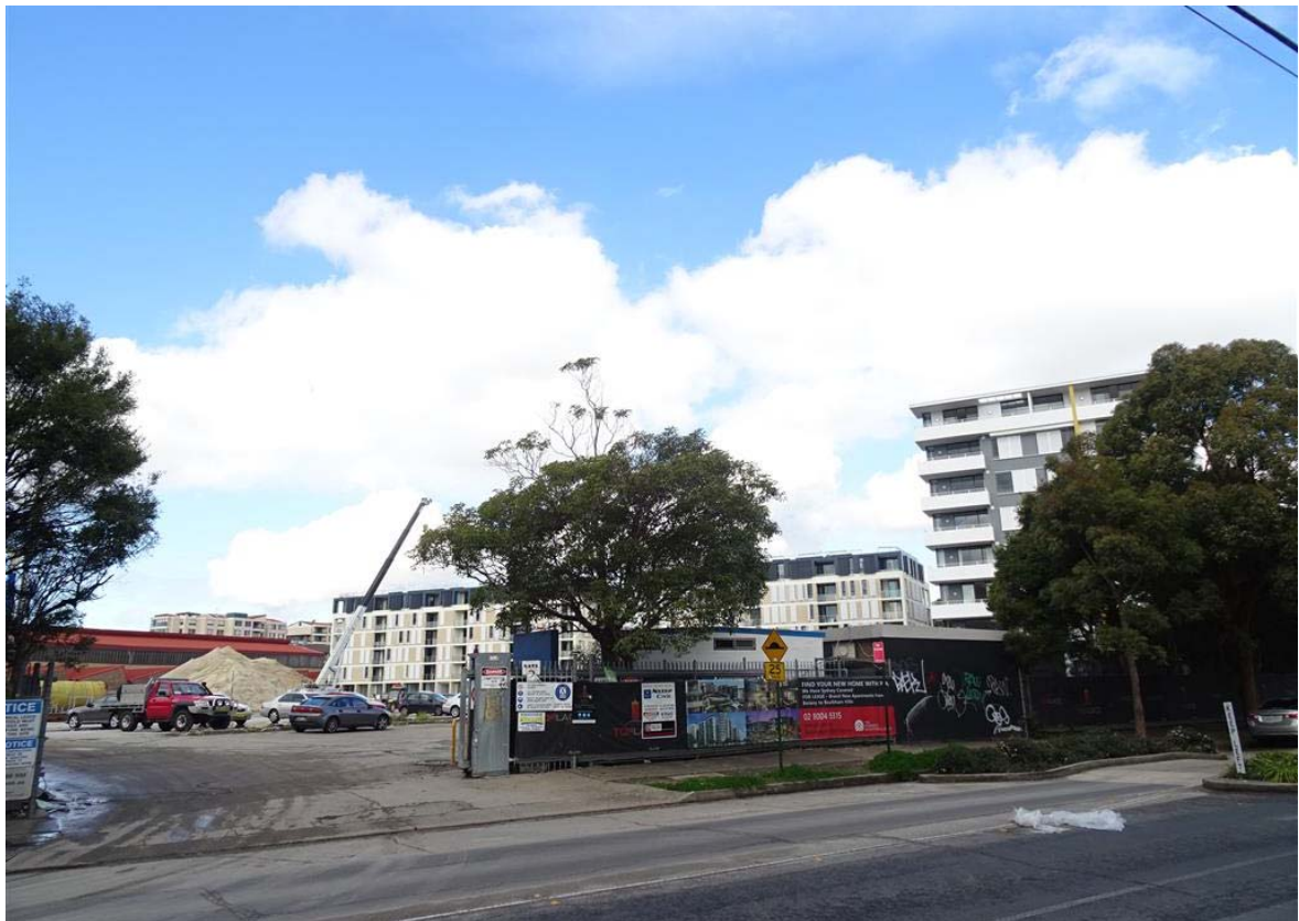
Figure 3: The site viewed from Dalmeny Avenue.
